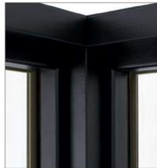
INTERIOR CLOSE UP
